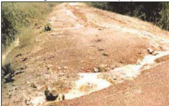
Figura A4-9 Surcos transversales (A4.6)
